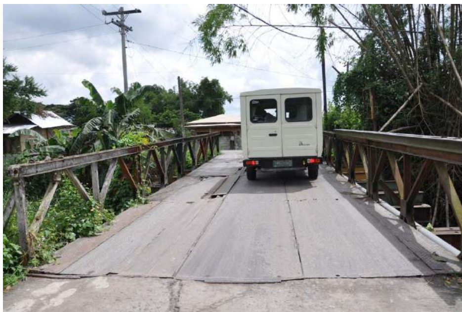
Figure 3.2.17. A View of the Deteriorating Laput Steel Bailey Bridge
