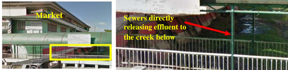
Figure 4-34 Effluent from Public Market Flowing Down a River
