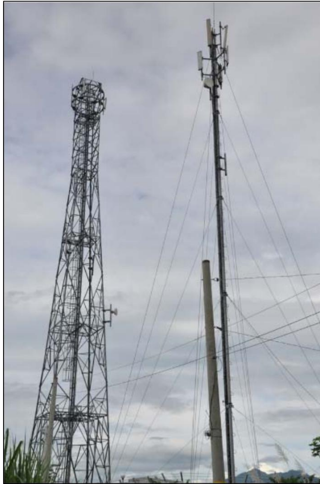
Figure 4-26. SMART Cell Site situated in Parian
