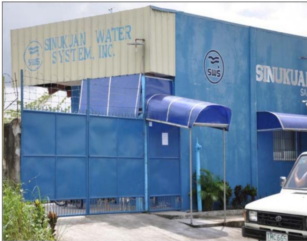
Figure 4-24 Sinukuan Water Pumping Station in Camuning
